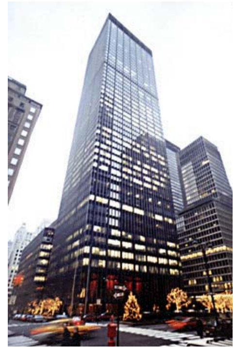
Ronsco recently completed work at the 1.1 million sq. ft. JP Morgan/Chase Building at 270 Park Avenue.
